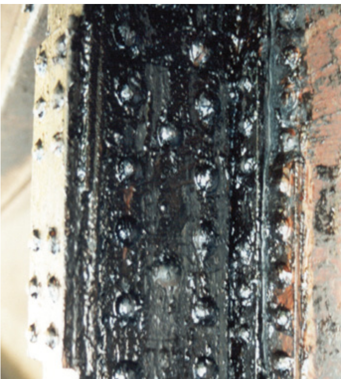
Removing resinated oil for renovation purposes
