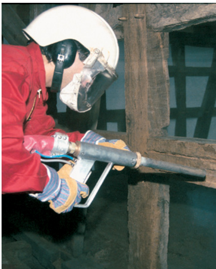
When dry ice blasting (e.g. when renovating an old half-timbered house, as shown here), always wear protective clothing.
